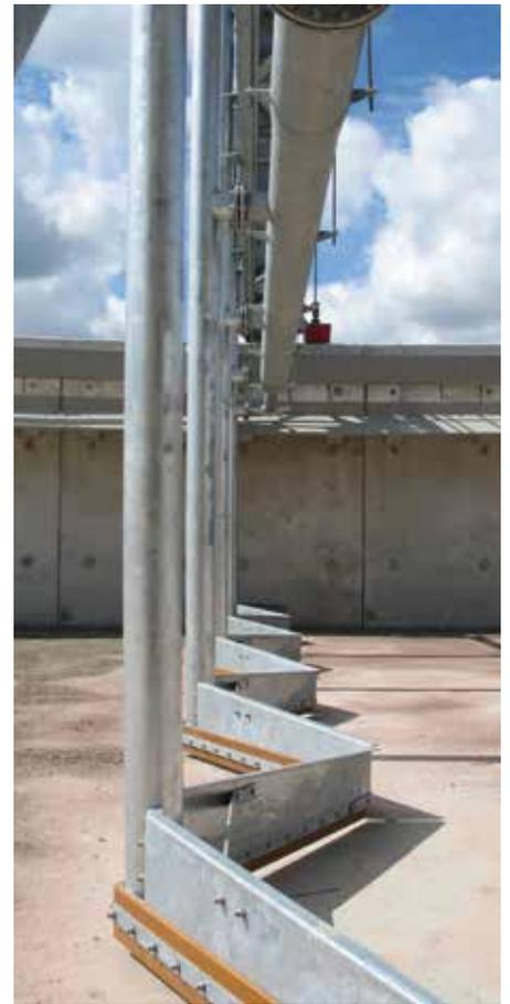
Suction-lift scrapers with suction down-tubes
