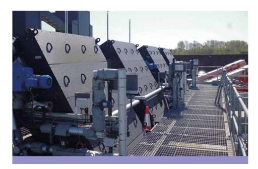
Each panel has a replaceable side seal manufactured from bearing grade ultra-high molecular weight polyethylene fitted between the chain and panel to effect a close tolerance seal, with the seal fitted to the screen structure.
